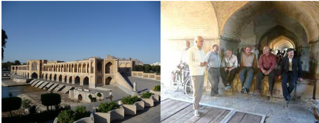
Fig. 2 Khajou Bridge of Isfahan, Iran
